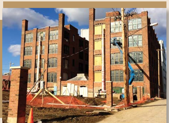
Carriage Factory Apartments
