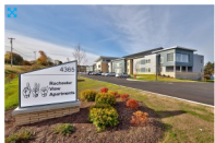
The $17.6 million DePaul Rochester View Apartments is designed for deaf and hard of hearing residents in Henrietta, N.Y.
