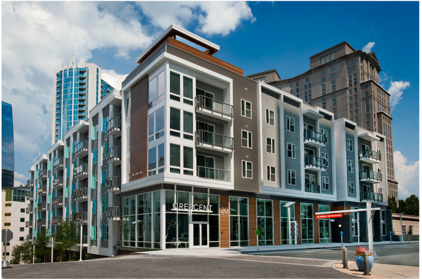
Crescent Terminus, a three-building luxury apartment community in the Buckhead section of Atlanta, was completed by Crescent Communities in 2014 and used wood-frame construction.
