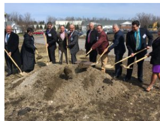
DePaul and civic leaders officials break ground for the new Apple Blossom Apartments on Old Union Road. (Jim Herr/Cheektowaga Chronicle)
