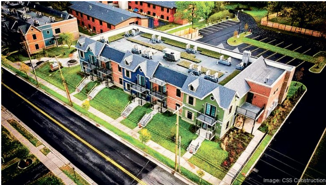
Blocher Homes in Williamsville CSS CONSTRUCTION
